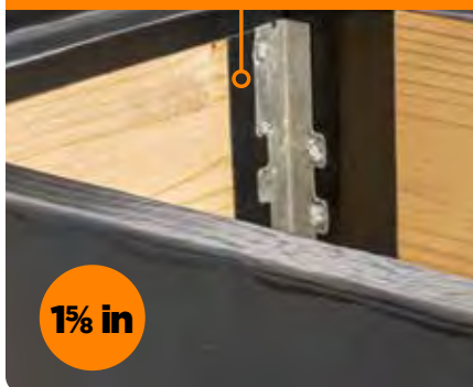
BETWEEN JOIST HANGERS AND LEDGER BOARD
