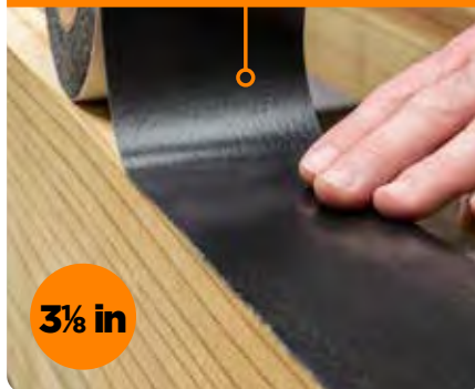
TOP OF DOUBLE JOISTS
