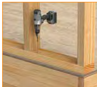
BOTTOM PLATE TO RIM BOARD
