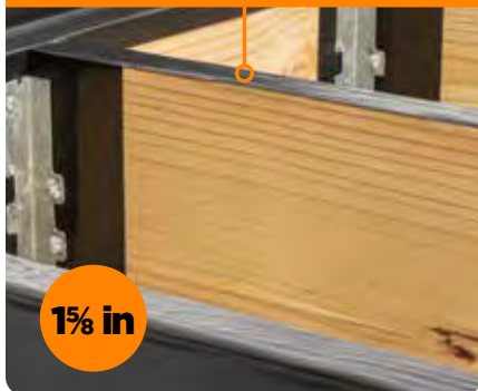
TOP OF JOISTS
