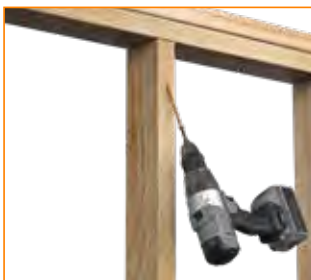
STUD TO DOUBLE TOP PLATE
