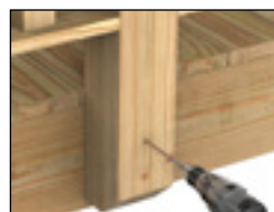
DECK POSTS, BEAMS + RAILINGS
