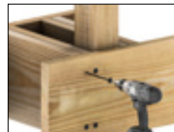
DECK POSTS, BEAMS + RAILINGS
