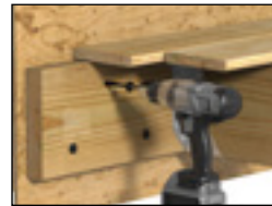
LEDGER BOARD CONNECTIONS
